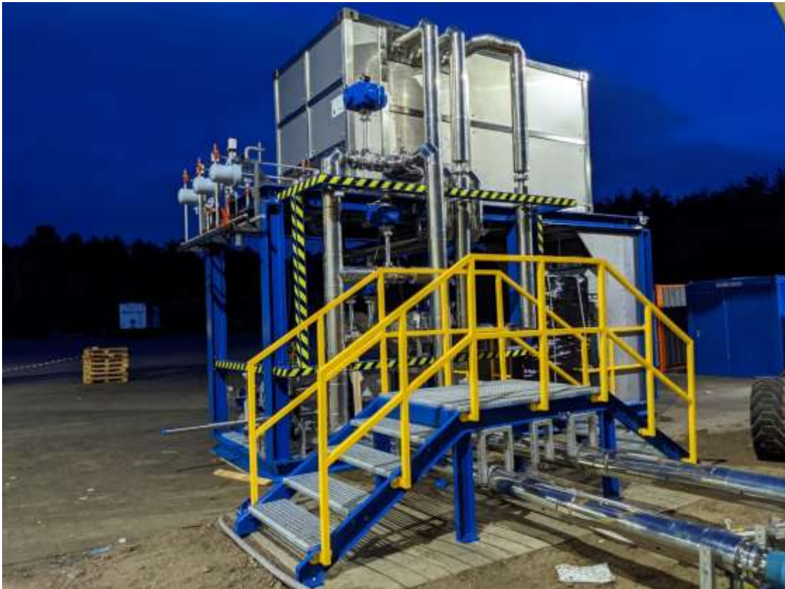
Figure 12. The skid and heat exchanger block connected and installed at Frigologix.
